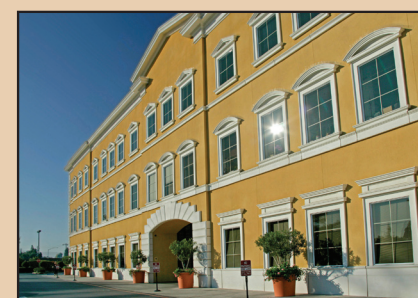
455 O'Connor Drive, San Jose 52,000 square feet
